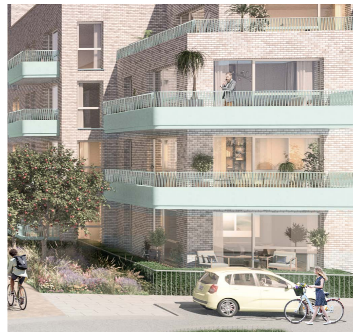
Figure 18: Block B1 wrap around balconies with chevron balustrades
