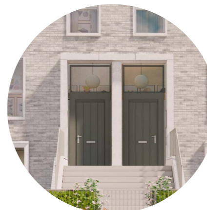
Concrete detailing to doors on duplex apartments
