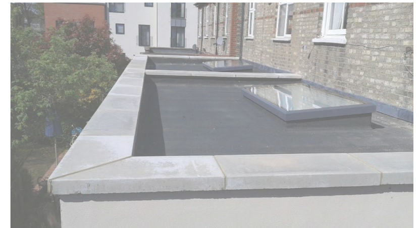
Concrete capping with effective drainage
