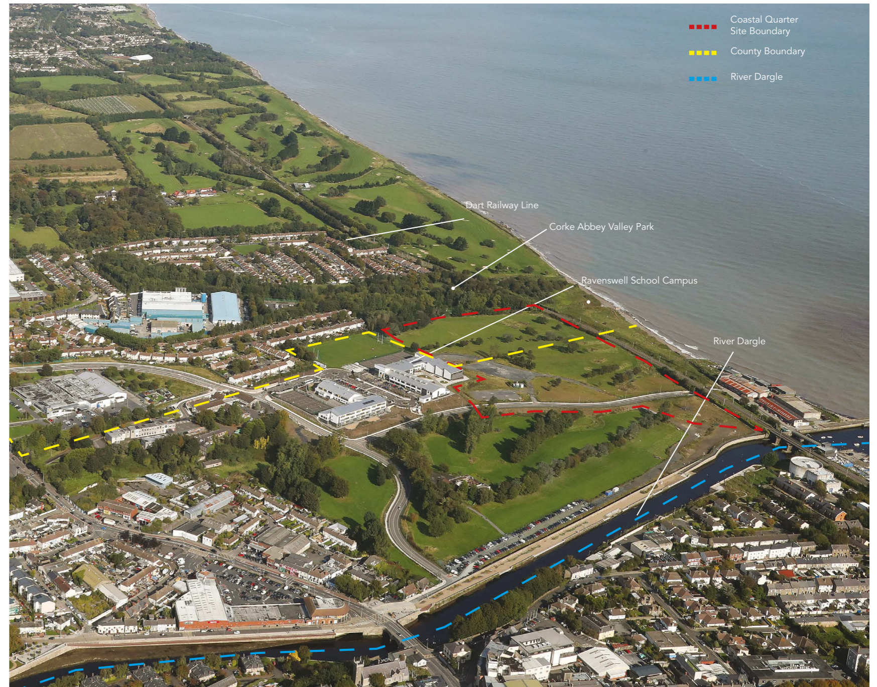
Figure 1: Aerial view of the site looking north towards Dublin Bay (Approximate site area outlined in red)
