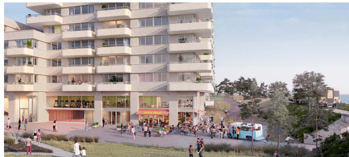
Figure 43: View showing connectivity to the Coastal Gardens and future connection to the existing Wicklow County Council path
