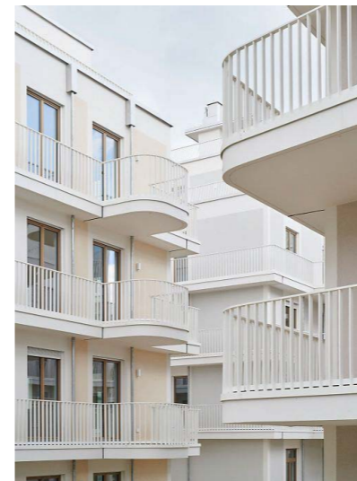
White banded brickwork
