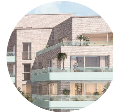
Every building has its own unique window detailing
