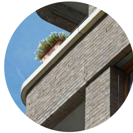
Caping profiles for drainage
