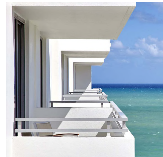
Solid upstand balcony with open top rails
