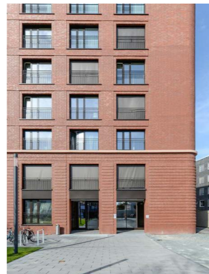
Bullnose Corner brick detail
