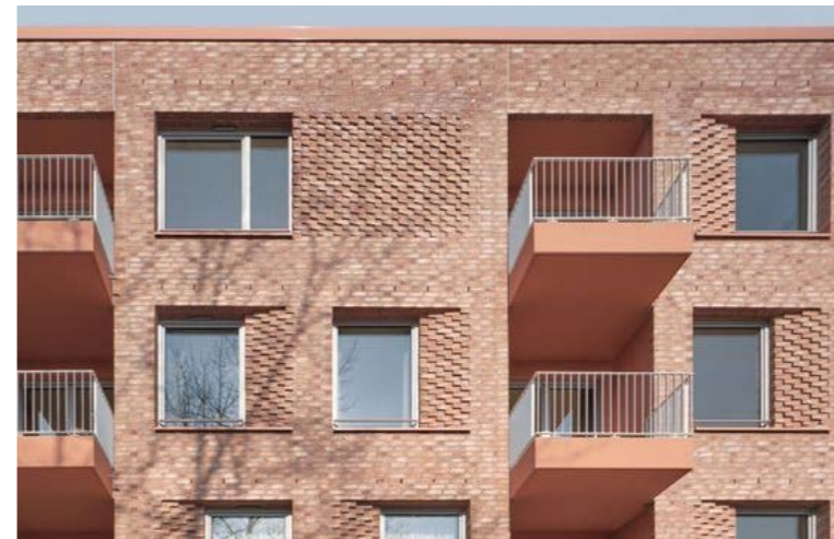
Confident brick facade wrap
