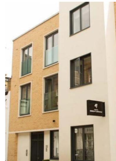
Glass barrier at window openings
