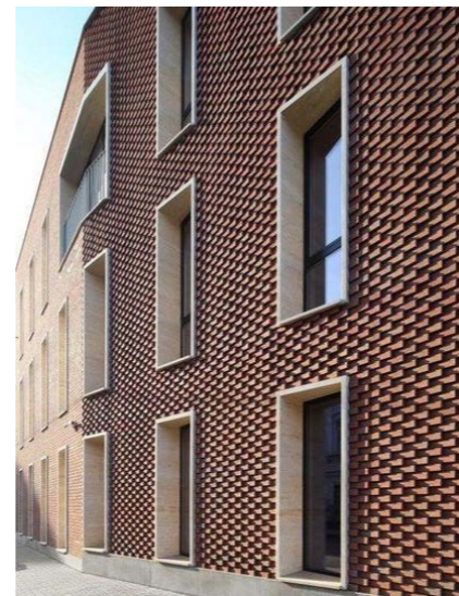
Concrete sills with overhang
