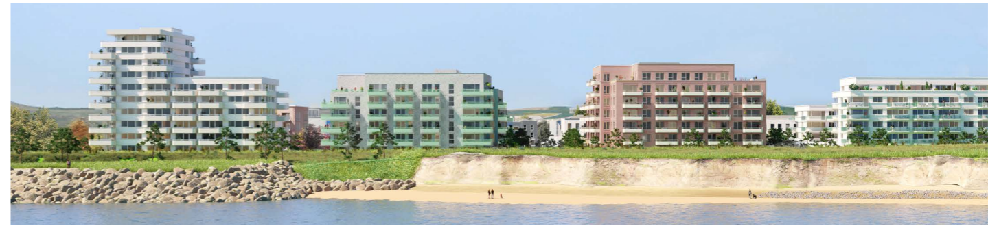
Figure 63: East elevation of Block A&B from the sea
